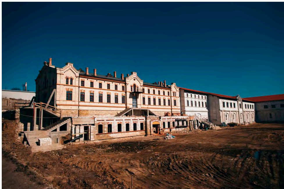
Fig. 5. Reconstruction of the wine-making complex from Bulboaca. Period of reconstruction works 2011-2016 7 .
